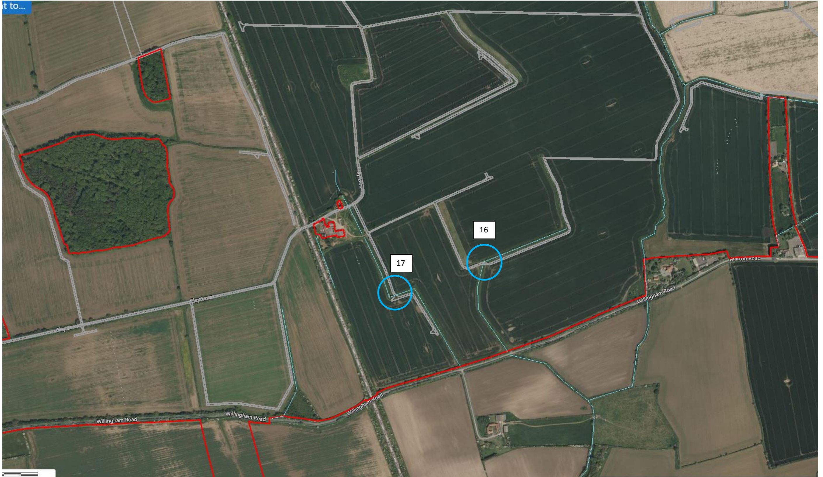
Solar and Energy Storage Park
